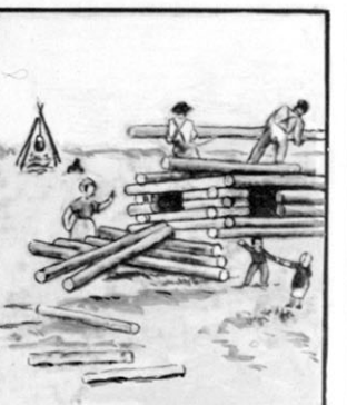
Building a house
